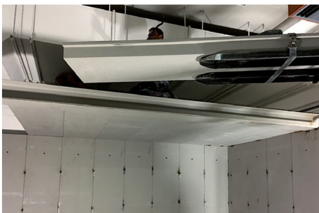
Installation of the ceiling panels
