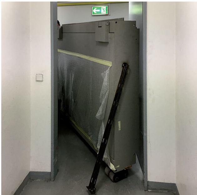
Transport of the vault door
